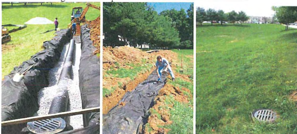
Figure 4: Example of Infiltration Trench Installation
